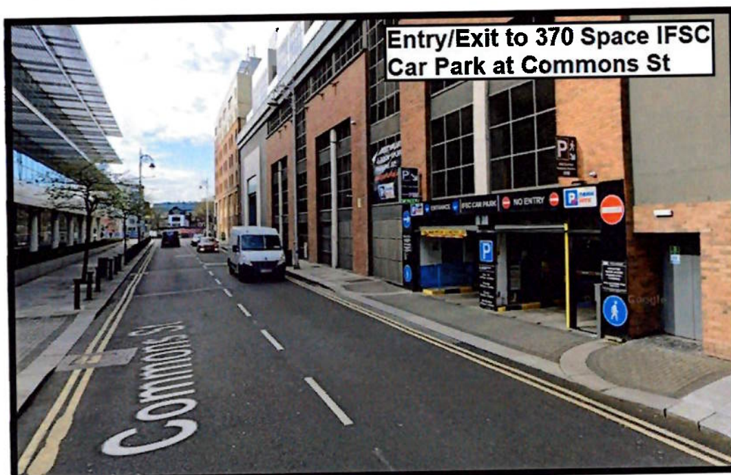
Figure 3.2: NRB Consulting Engineer's annotated Google Streetview image showing Commons Street IFSC Carpark.
